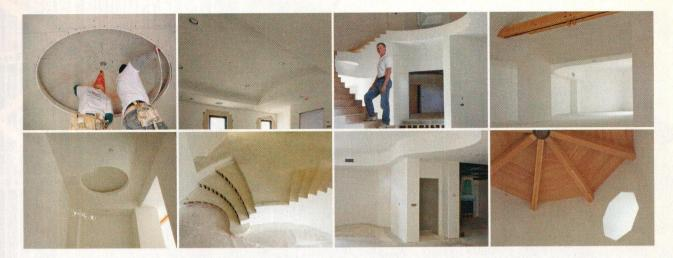
Off-angles were coved using Select Taping Tools' Off-Angle Head.
